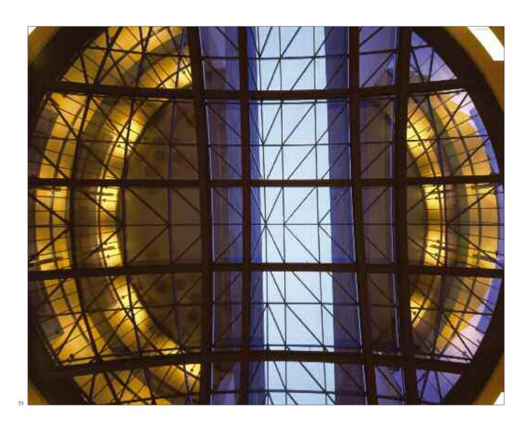
53. The dome over the atrium: a convex and circular skylight made of steel and glass.
