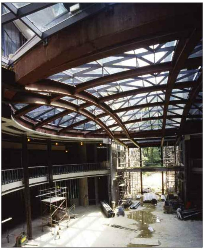
61. Stages of construction: the reticular structure of the central atrium dome with its triangular mesh of steel bars and glass plates.
