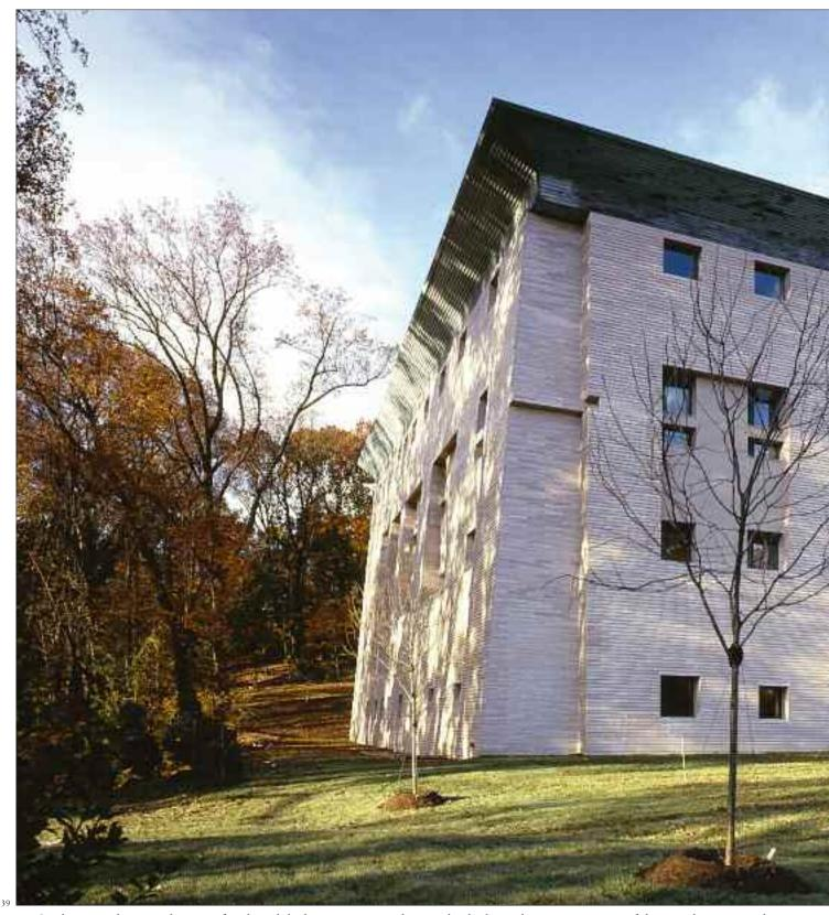
39. On the corner between the major façade and the buttress, a stone element clearly shows the interconnection of the two planes, vertical and inclined.
