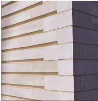
Architect P. Sartogo watching the rosa Asiago stone elements that he conceived as soft skin enfolding the entire building. The stone modules dimensions are 60 cm in length, 12 cm in height and 10 in depth. They have a side cut with an inclination of 45 degrees to outline the horizontal superimposition of layers.
