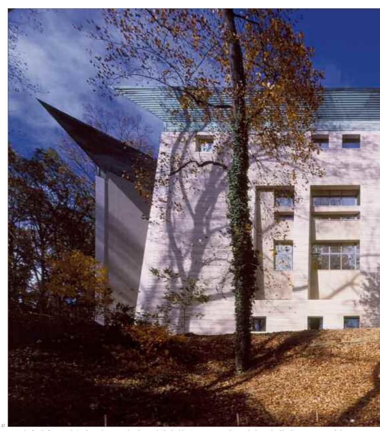
17. In the façade facing Rock Creek, nearly immersed in the woods, the building's mass counters the steeply sloping land by the incorporation of a buttress.
